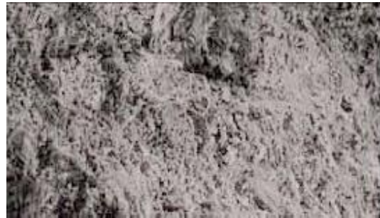
concrete after treatment with DRS-FLOOR HDP
